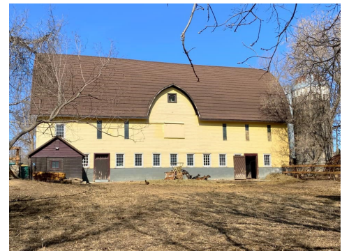
Photo by Katie Sherva Carsi Barn in Hennepin County
