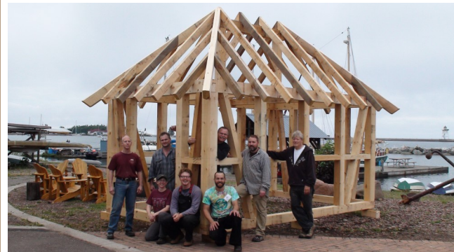
North House 'German style timber framing' class
