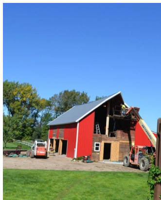
2016: start of renovation process
