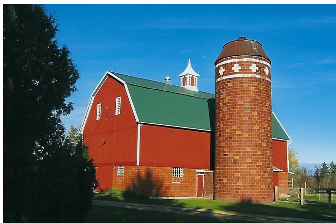
2009—same barn as above with new roof, fresh paint and cupola restored
