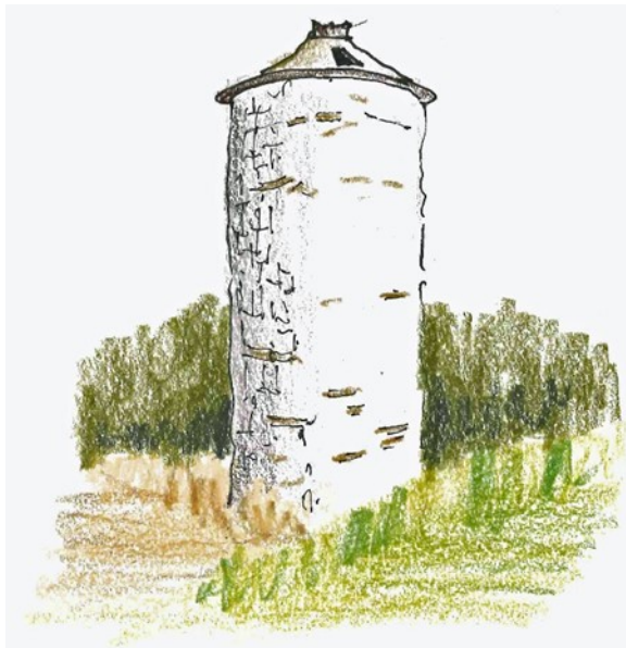
A freestanding stone silo covered with deteriorating white painted cement plaster parging. Wolf Creek, Wisconsin.
